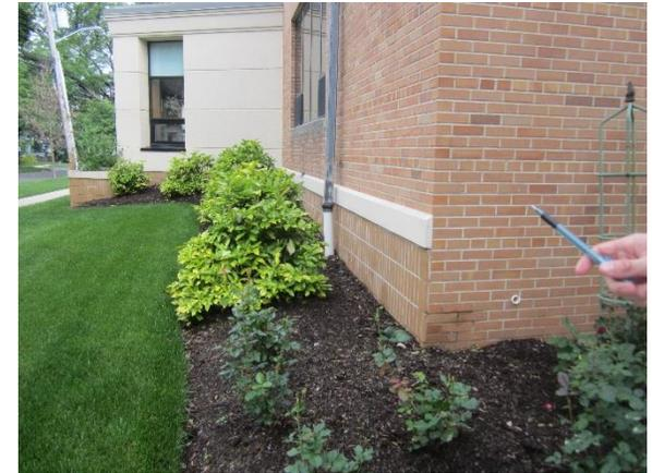
A downspout can be disconnected and directed into a bioretention system near the corner of 3rd Avenue and Summit Place, which will capture, treat and infiltrate roof runoff. A preliminary soil assessment suggests that more soil testing would be required before determining the soil's suitability for green infrastructure.
