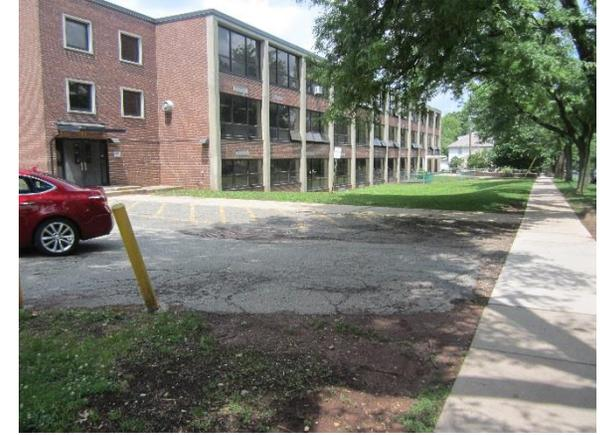
Several areas can be converted to porous pavement to infiltrate runoff. Downspouts on the southern end of the building can be disconnected to allow stormwater to infiltrate into an existing turf grass below. Another downspout can be disconnected a cistern to harvest rainwater, and a rain garden on the eastern side of the building can capture, treat, and infiltrate runoff. A preliminary soil assessment suggests that the soils have suitable drainage characteristics for green infrastructure.
