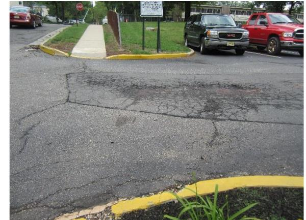
Parking spaces next to the building can be repaved with porous asphalt to infiltrate runoff. A preliminary soil assessment suggests that the soils have suitable drainage characteristics for green infrastructure.
