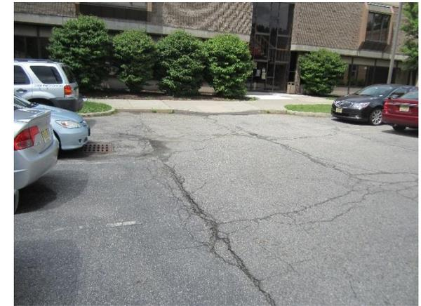
Parking spaces and a portion of the sidewalk can be repaved with porous pavements to infiltrate stormwater. A rain garden can also be installed to capture, treat, and infiltrate runoff. A preliminary soil assessment suggests that the soils have suitable drainage characteristics for green infrastructure.
