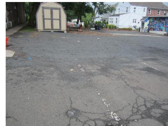
A portion of the parking lot can be repaved with porous asphalt to manage stormwater. The optimal locations for this porous asphalt would be uphill of three existing catch basins. A preliminary soil assessment suggests that the soils have suitable drainage characteristics for green infrastructure.
